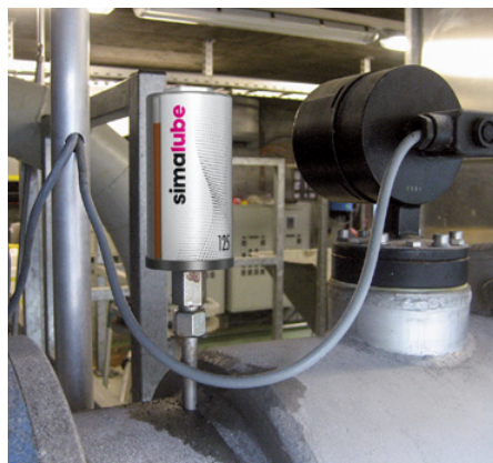
Lubricating bearings: the lubricant is transported to the bearings via a short pipe.
