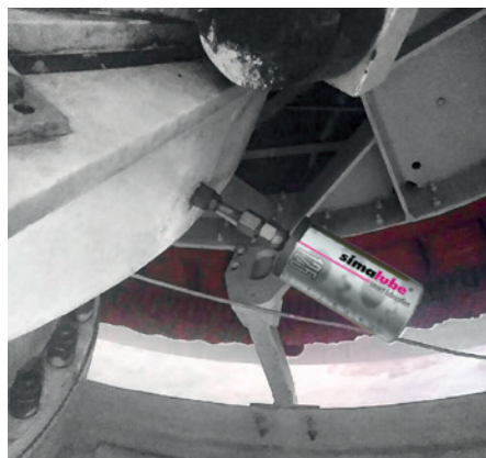
In this wind turbine, the simalube lubricator is set with a dispensing time of six months.
